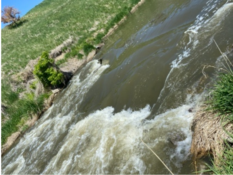
Figure 38. Tailrace Hydrologic Jump near the spillway
