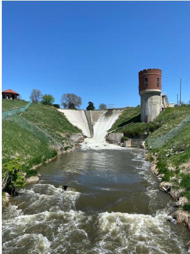
Figure 39. View of the Tailrace Site looking towards the Spillway
